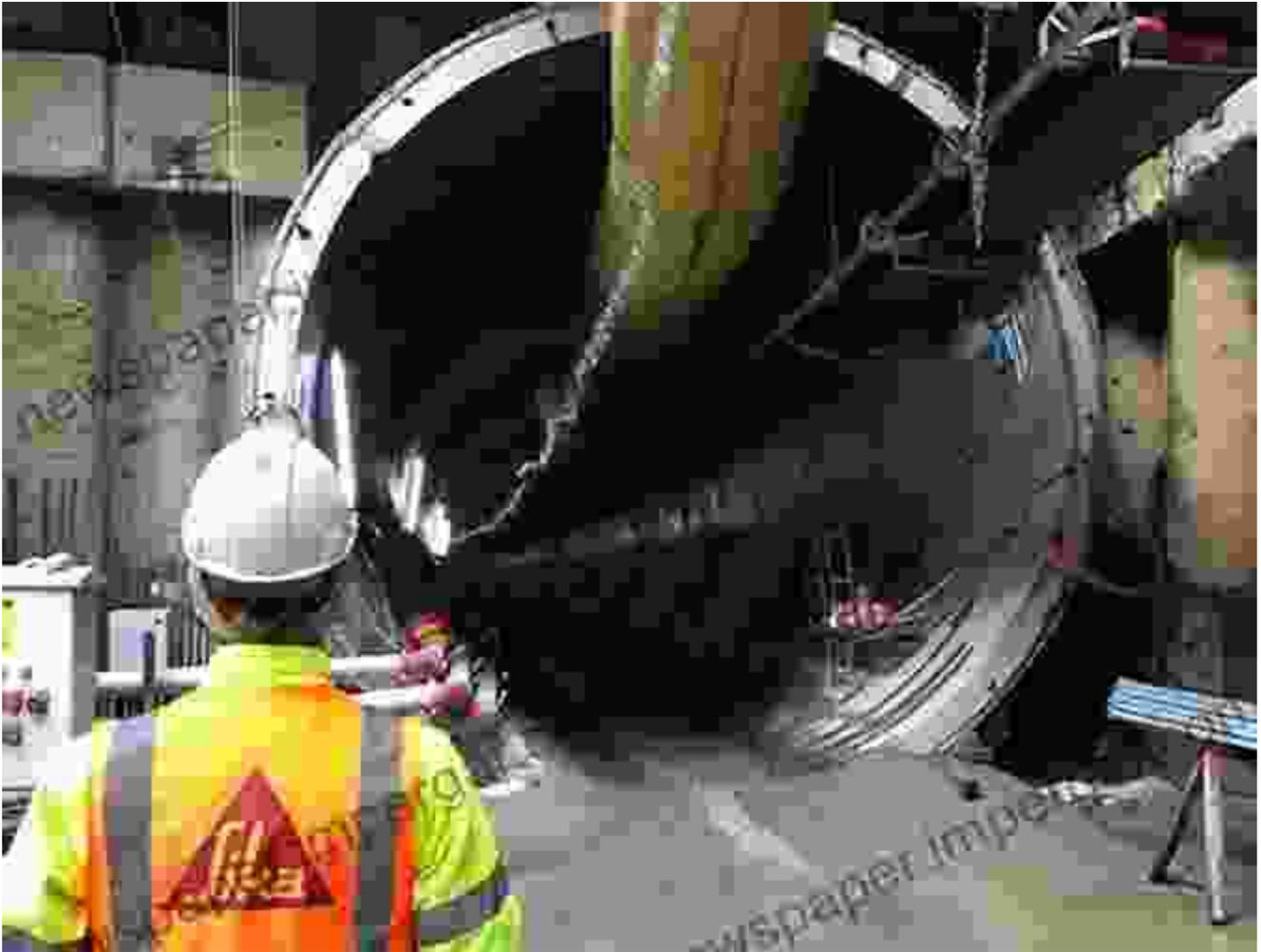
The shield itself consists of a cutting head, a main body, and a tail seal. The cutting head rotates to excavate the soil, while the main body houses the hydraulic jacks that push the shield forward. The tail seal prevents water from entering the tunnel.
